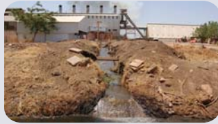
Industrial waste water disinfection
